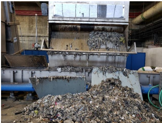
Figures 7 and 8: Back sides of the bar screens, opened to remove screenings (instead of using the sluice).
