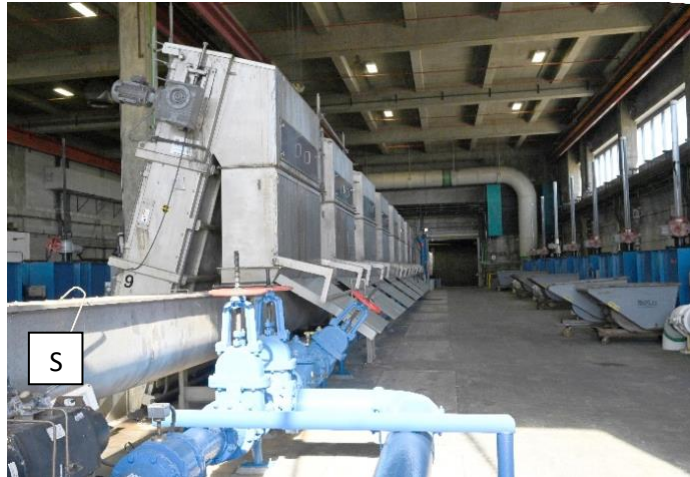
Figure 2: Array of eight Hyperion bar screens, sluice marked with S.
