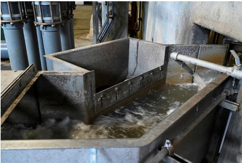
Figure 14: Sluice showing emergency overflow weir, sluice continues through the wall to chopper and spiral lifts.
