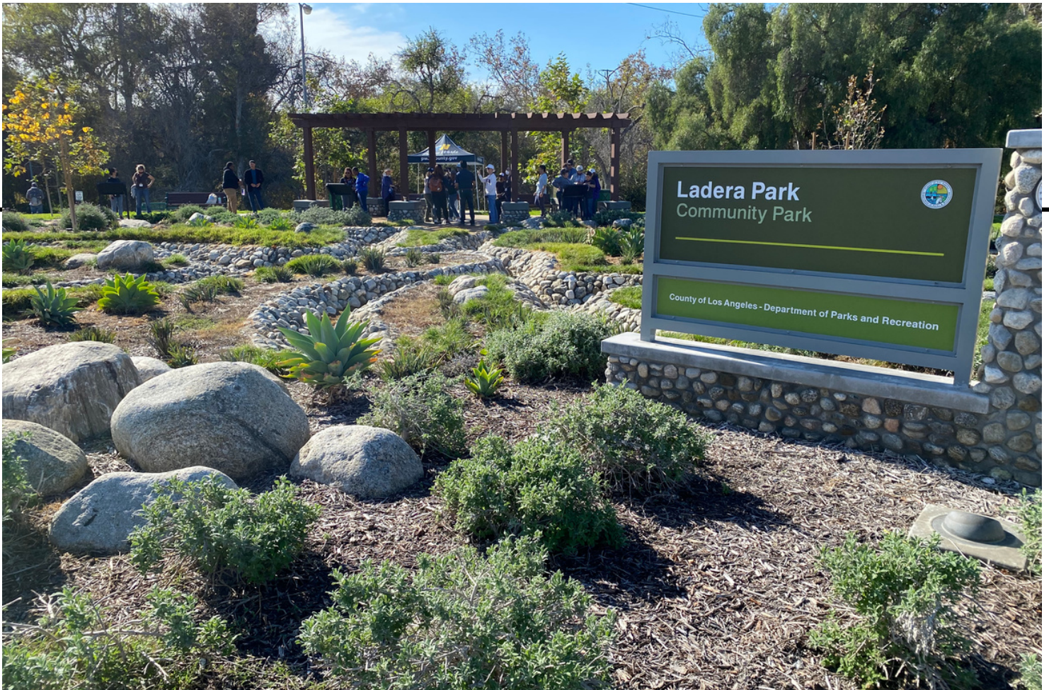
Ladera Park Stormwater Improvements Project: multi-benefit stormwater capture project offering improved water quality, onsite use and infiltration of stormwater, enhanced recreational and educational opportunities, and more. Photo by: Heal the Bay.
