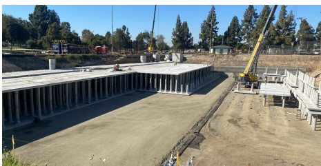
Adventure Park Multi Benefit Stormwater Capture Project: stormwater capture project with an infiltration gallery, funded by the Safe, Clean Water Program. The project is shown here under construction (far left and far right), and ensuring proper tree protection (center). Photos by: Heal the Bay.
