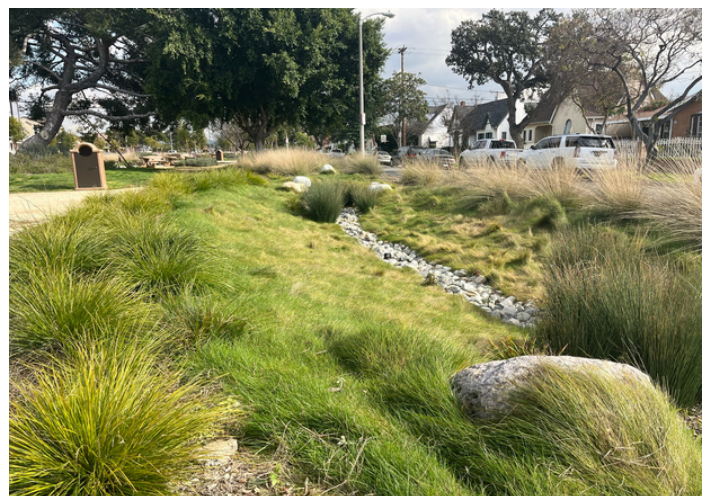
East Los Angeles Sustainable Medians Project: multi-benefit stormwater capture project offering flood protection, water quality improvements, recreational opportunities, increased shade, enhanced habitat, and more. Photos by: LA Waterkeeper.
