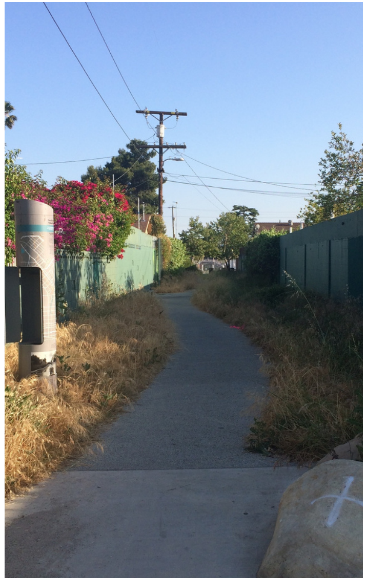
Elmer Avenue Neighborhood Retrofit: green alley with permeable pavement, climate-appropriate vegetation, and infiltration galleries. Photo by: Heal the Bay.
