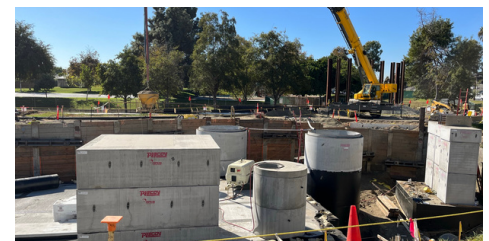
Adventure Park Multi Benefit Stormwater Capture Project: stormwater capture project with an infiltration gallery, funded by the Safe, Clean Water Program. The project is shown here under construction (far left and far right), and ensuring proper tree protection (center). Photos by: Heal the Bay.
